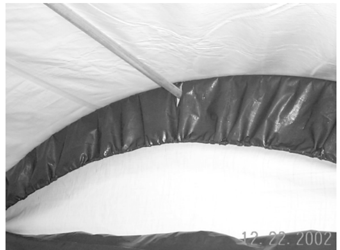
End Panel / Doors have pre-cut slots that allow Cross Rails to pass through, so material can wrap around arch with rope pocket inside unit
