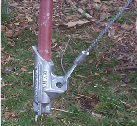
Drive Rod inserts into Anchor Head
