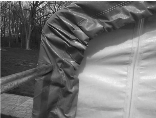
**Note:** Snug the end panel by turning the turnbuckles or repeating step 3 on a regular basis
