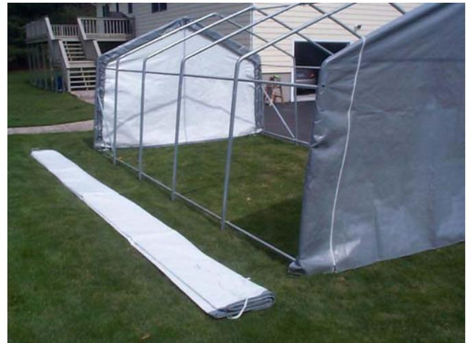
Once cover is oriented properly to the Frame Assembly, pull Main Cover over frame assembly from the side, being careful not to snag the cover on any member, bolt, or other obstruction. Center the Main Cover over the Frame Assembly with the Main Cover colored side showing from the outside of the unit.
