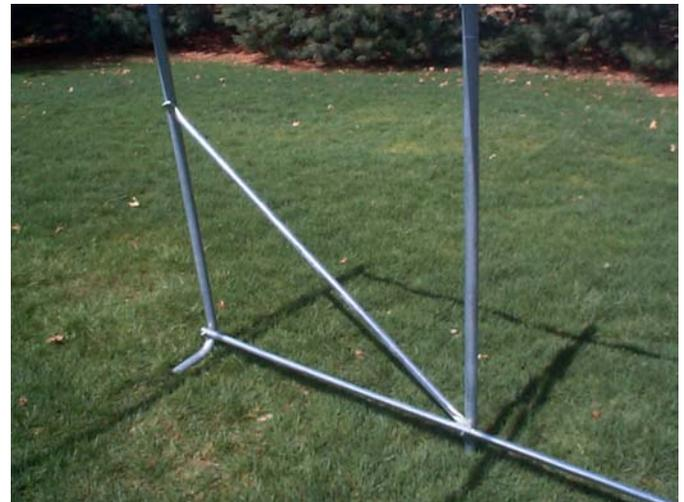
**Step 6.** Add remaining 3 middle arches and rear end arch in the same fashion. Use SCR-2004 Cross Rails for each connecting base, ridge, and top rails. The swaged end of the cross rails should be inserted into the prior end rail at all arches. Note that the Ridge Crest Rail should fasten under the End Top Crest Arches but above middle Top Crest tubes.
