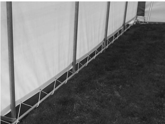
Pay close attention to how tight the cover is put onto the frame. It should be tight enough so it does not flap
