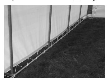
**Step 4.** Retighten or readjust the turnbuckles on both the cover and end panels as needed. Retighten the rope holding the main cover to the bottom cross rail. **Both the cover and the end panels should be checked and tightened on a monthly basis.**
