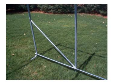
**Step 5**. Begin the Top Ridge Rail by placing the final ECR-2031 Plain End Cross Rail <u>underneath</u> the End Arch Tube. Secure the Cross Rail loosely with a Carriage Bolt CBN-3000-3 with washer and nut facing the interior of the unit. This begins the Top Ridge Rail. The other end of the Cross Rail goes on top of the Interior Arch as shown in the illustration.
