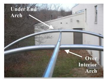
**Step 7**. Move the frame assembly into its final installation location. This should be done with at least two people lifting each arch upright and corner to avoid bending or stressing any frame members.
