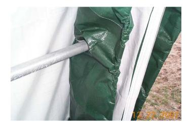
When putting on the doors, adjust the length to make certain the doors do not drape onto the ground. If pulling them up puts too much stress on the slit where it goes over the wind brace, use a sharp knife to cut slit another inch or two to relieve it. The PE fabric is rip-stop weave, and can easily be cut to relieve stress at the frame members.
