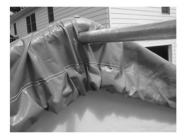
The rope channels should be located inside the unit, with the frame members passing through the pre-cut slits in the end panel/door. Replace and tighten the carriage bolts after putting the end panel into position.
